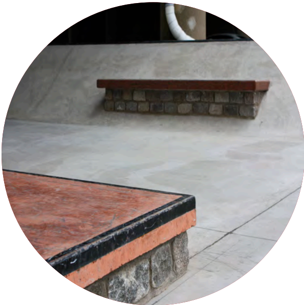
Figure 16. Stone ledge features integrated into a concrete walkway. Photo: New Line Skateparks
